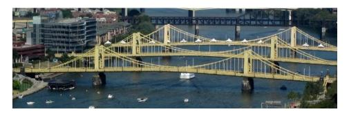
The Three Sisters are three similar self-anchored suspension bridges spanning the Allegheny River and connecting the North Shore to downtown.
